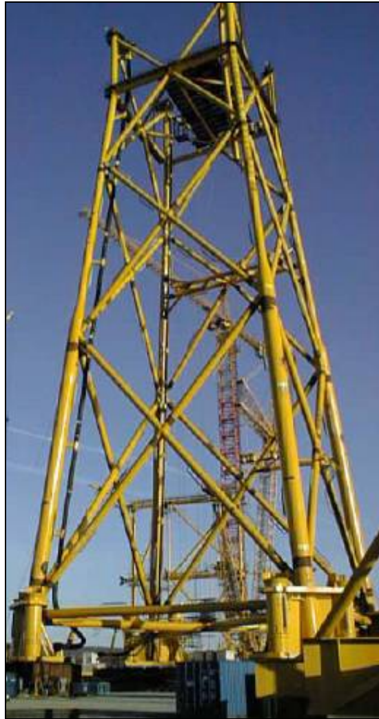
Figure 1 - Steel jacket for the North Sea at Aker (illustration photo of earlier similar project)
